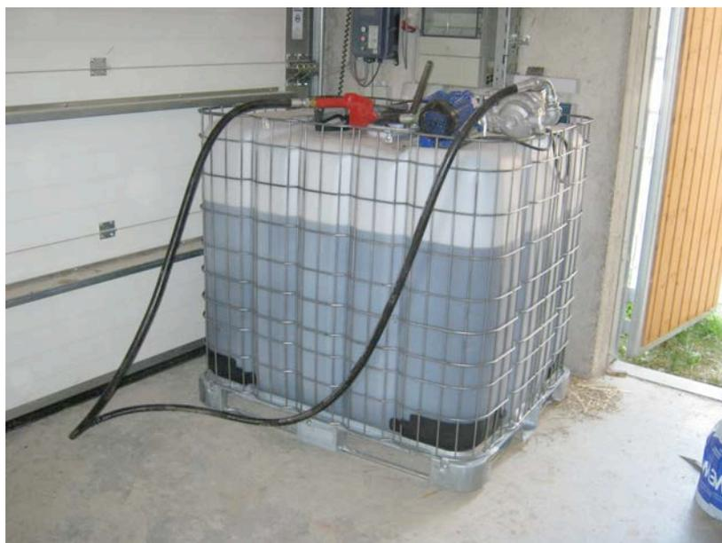
*Illustration 5: Biodiesel-pump system (1000 litres IBC), Josef Koller – Gersthofen*
